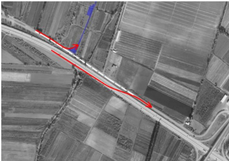
Figure 5-5 Access Point No. 1. Entrance to T03, T09, T19, T32
