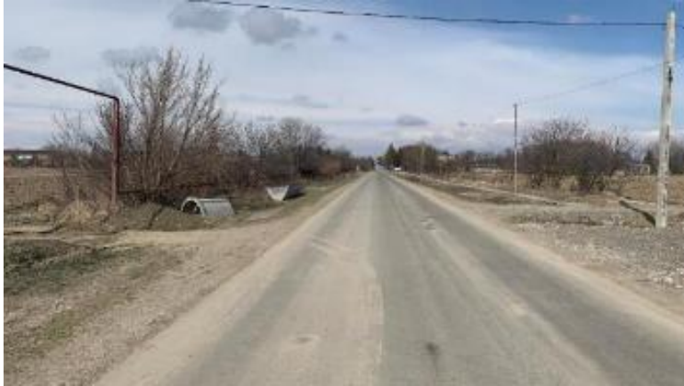
Figure 5-12 Gas pipeline to be rebuilt
