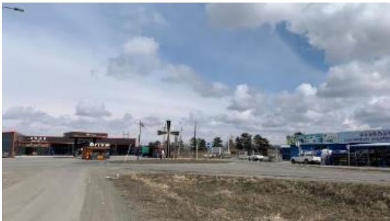
Figure 5-10 Roundabout in need of hardening
