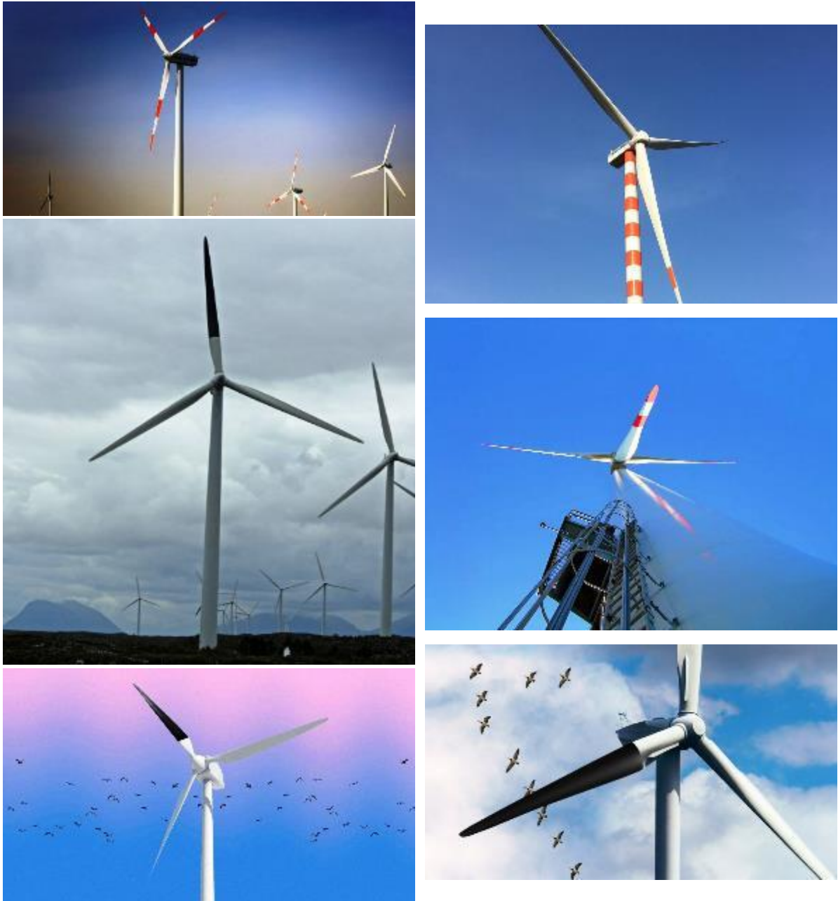
Figure 6-42 Marking of wind turbines with luminescent paint
