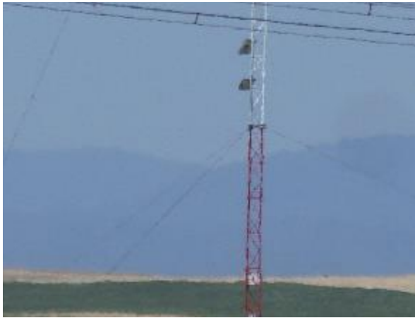
Plot 5. Wind Turbine #20. Wind metering pylon
