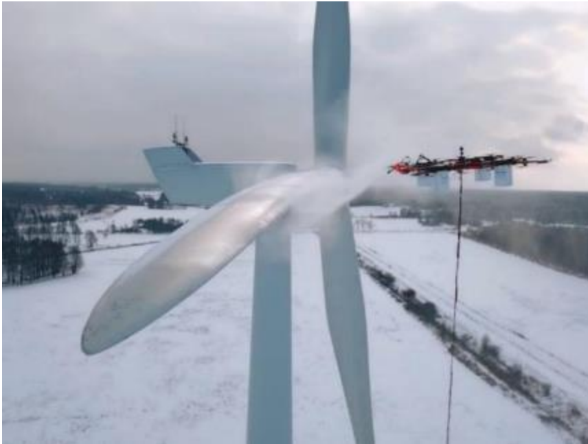
Figure 6-56 Use of the drone for cleaning of the wind turbine
