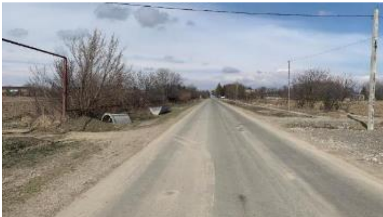
Figure 4-11 Gas pipeline to be rebuilt
