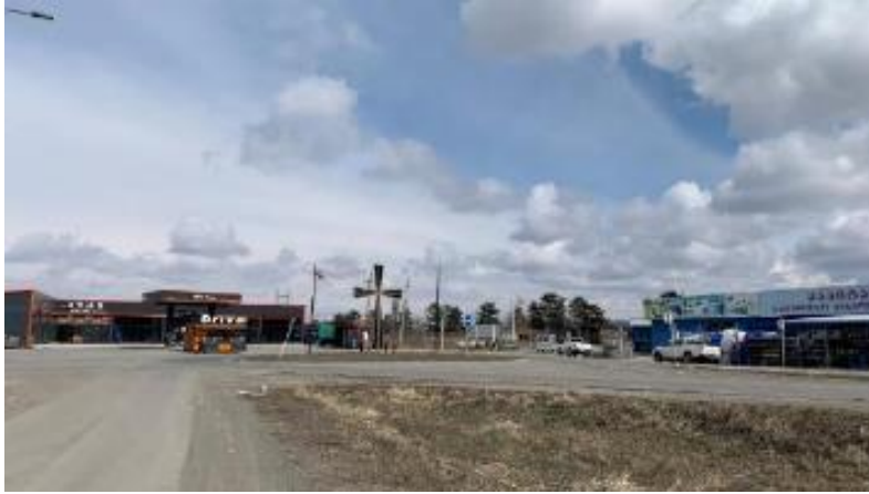
Figure 4-9 Roundabout in need of hardening
