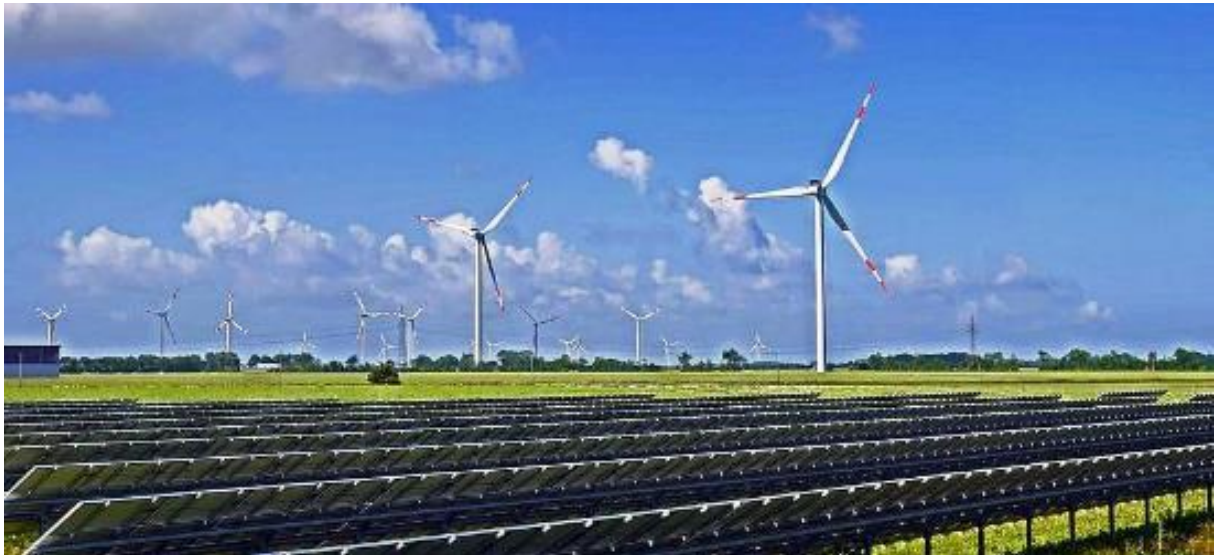
Figure 6-41 Marked wind turbines at the wind farm.
