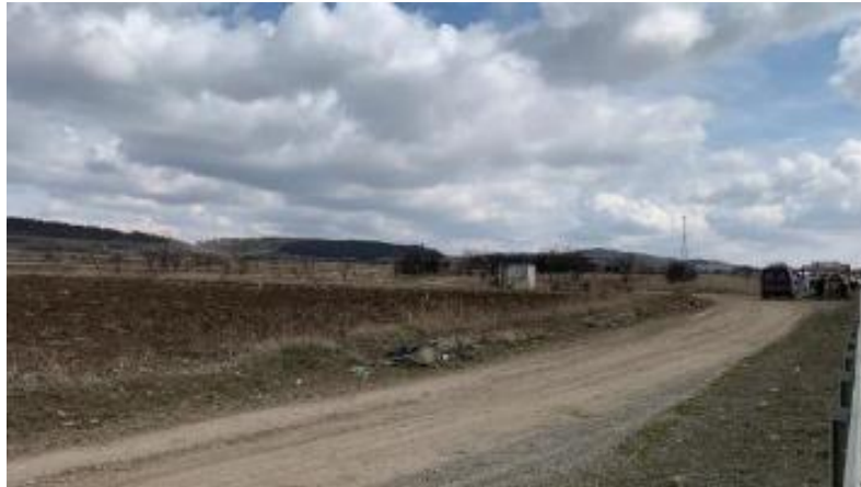
Figure 4-15 Access point 3. Road in need of reconstruction
