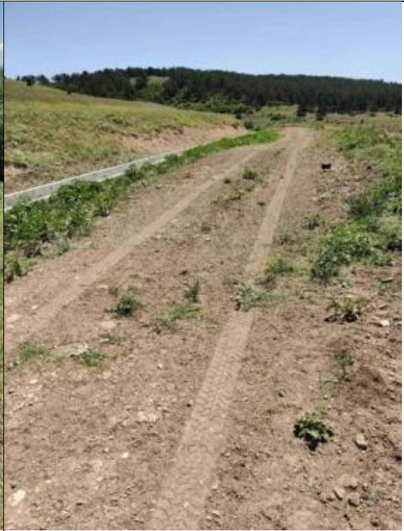
Photo 6 (Site I) ground fill along the irrigation channel under construction
