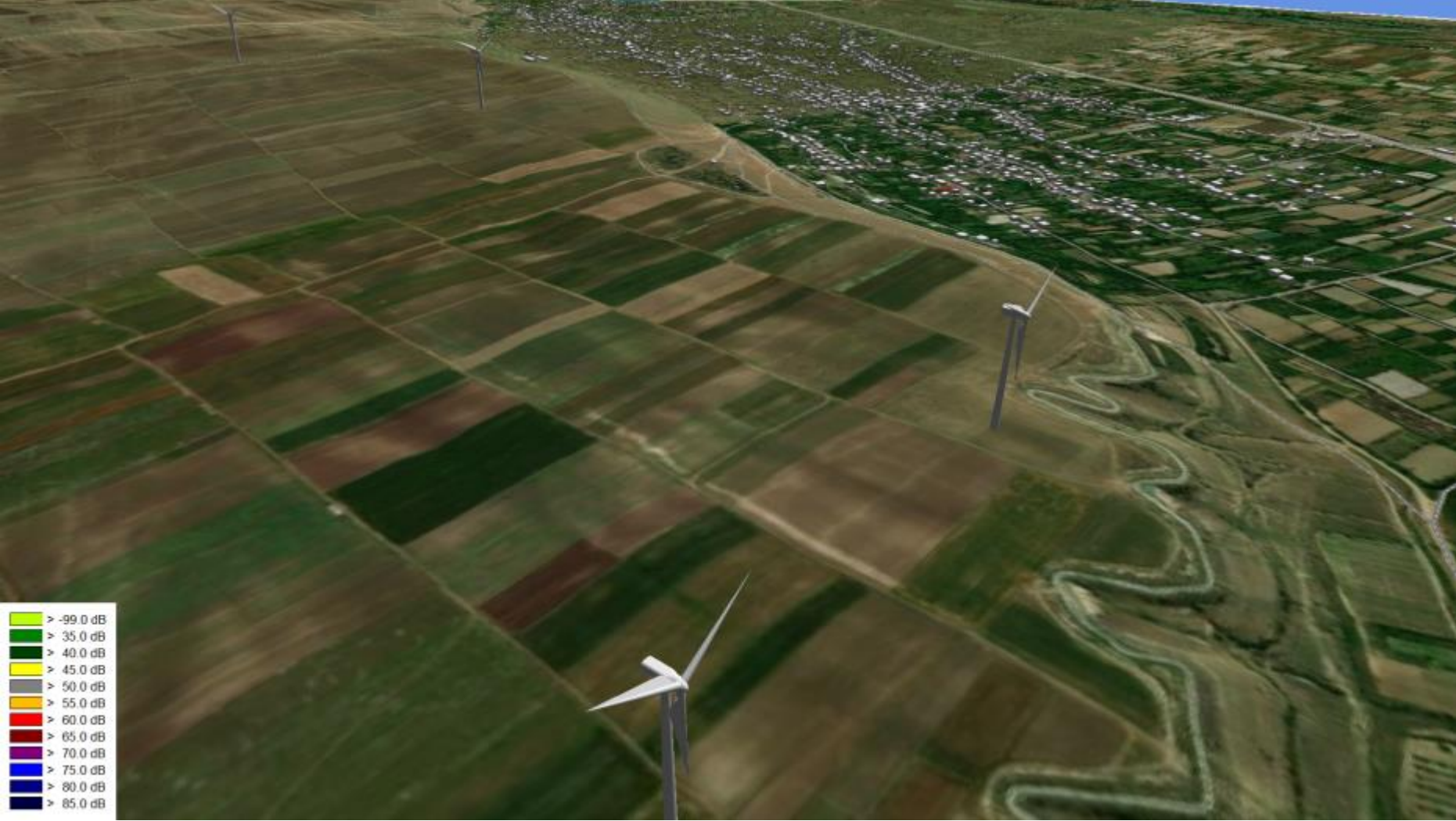
Figure N9.2: Initial view of the project area
