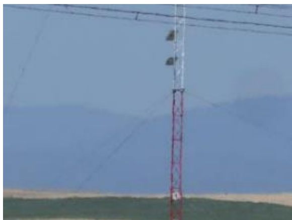
Plot 5. Wind Turbine #20. Wind metering pylon
