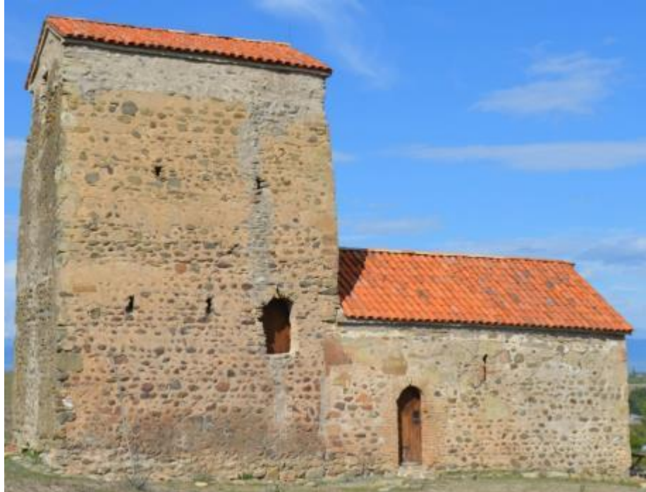
Tsveri Complex (church and tower)
